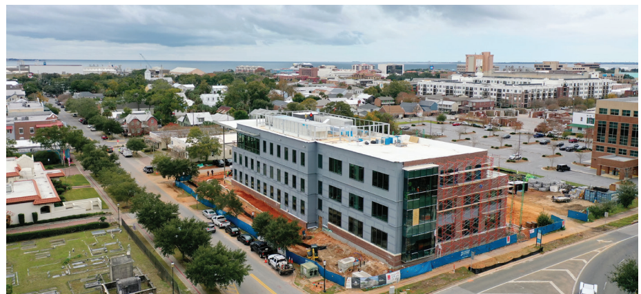
A view of the construction site from October 2023
