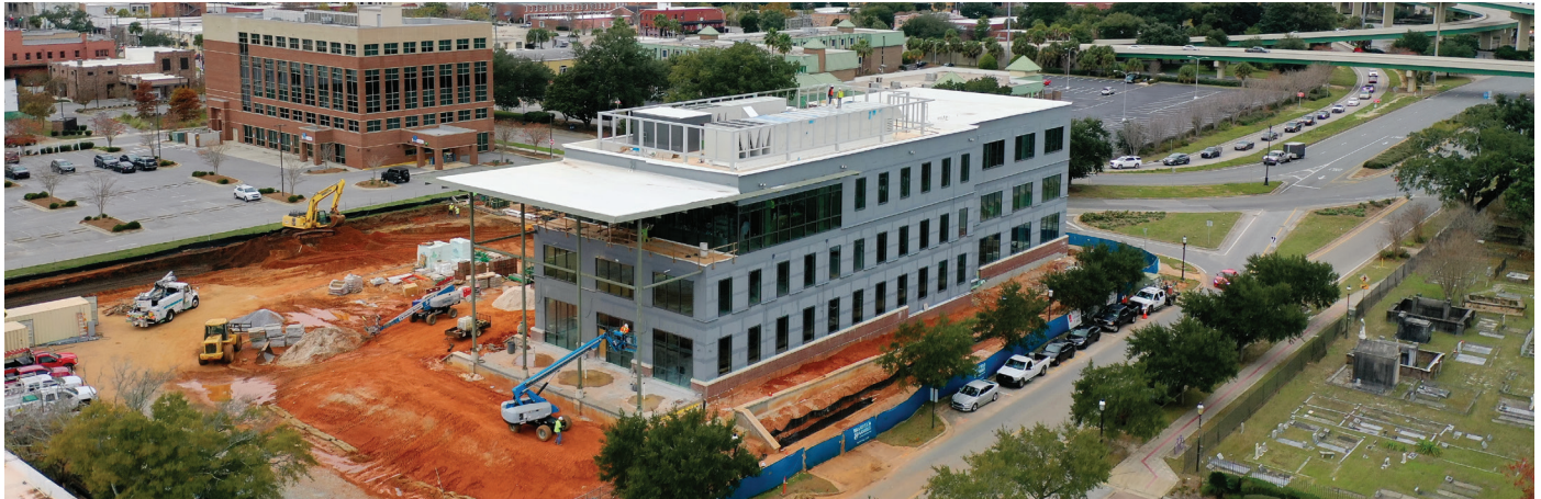
A view of the construction site from October 2023
