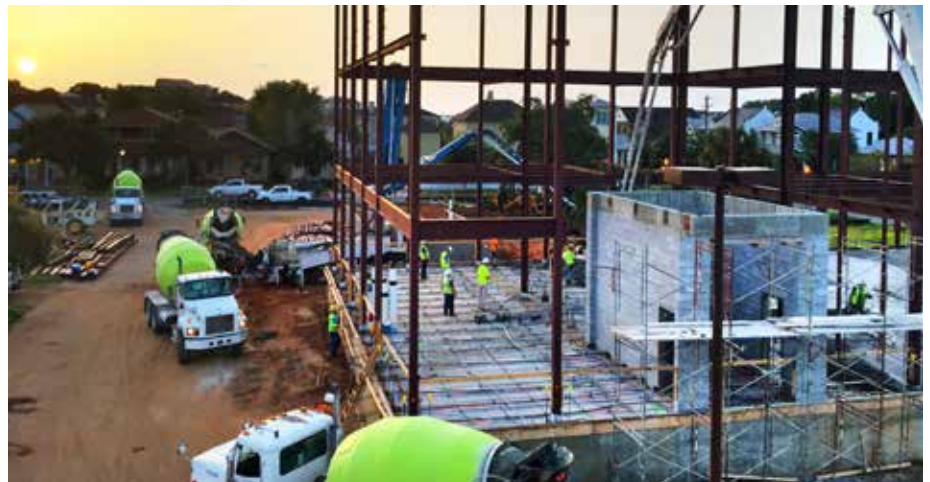
Crews arrived before sunrise to pour the first-floor concrete slab
